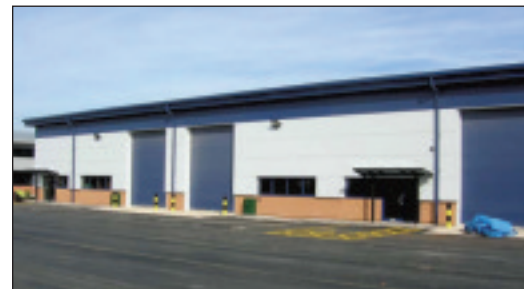
Brand New Units Bentley Business Park, Dinnington
