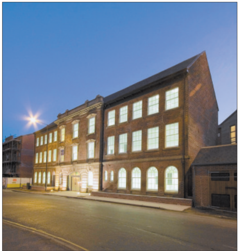
Kelham House on Neepsend Lane has been refurbished at a cost of £1m
