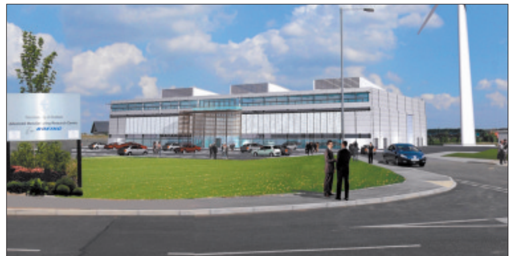
Futuristic: Part of the Advanced Manufacturing Park being built in Sheffield
